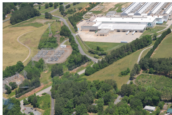
Edge of Alcoa-Badin Landfill and location of Outfall 005, which has had over 20 water quality violations for cyanide and fluoride since 2019
